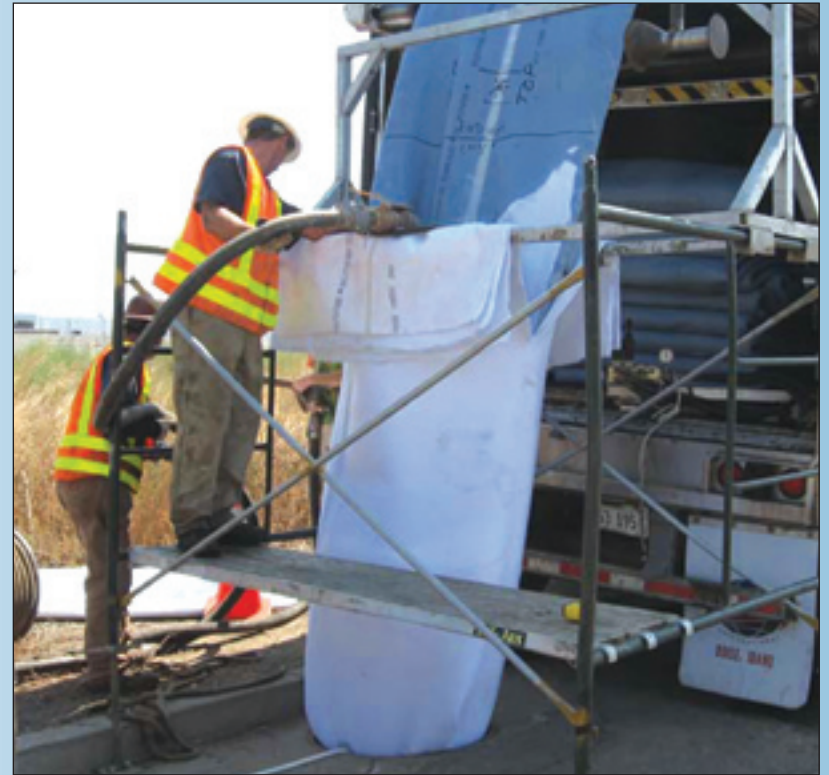
Inverting a 36” diameter liner from refrigerated truck
