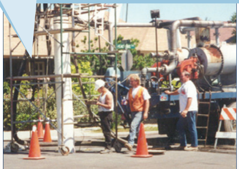
Curing or hardening the liner tube through circulation of hot water.
