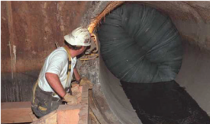
View of Pipeline with liner tube being “inverted” into host pipe.
