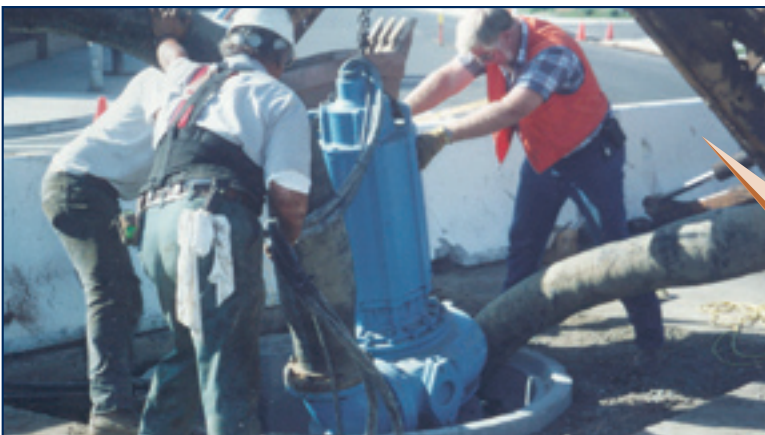
Bypass Pumping: Installation of submersible pumps at manhole.
