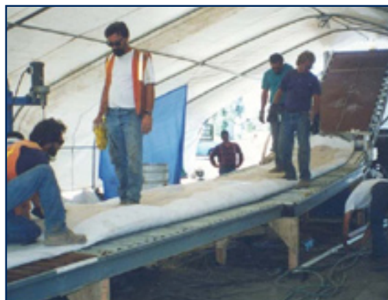
Saturating liner tube with resin inside a tent
