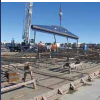
Construction on the LEED-Certified building began in 2007.
