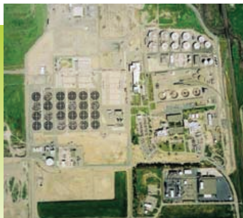
Aerial View of the Sacramento Regional Wastewater Treatment Plant
