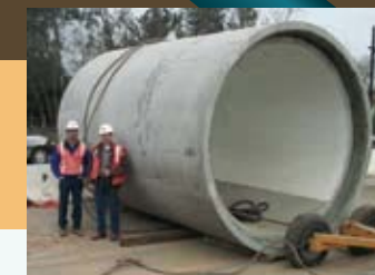
An interceptor is a large pipe – from 36 to 144 inches in diameter – that receives wastewater from smaller pipes throughout the region and conveys it to the wastewater treatment plant in Elk Grove.
